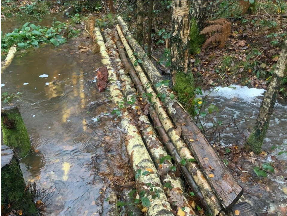
Leaky dam in action
