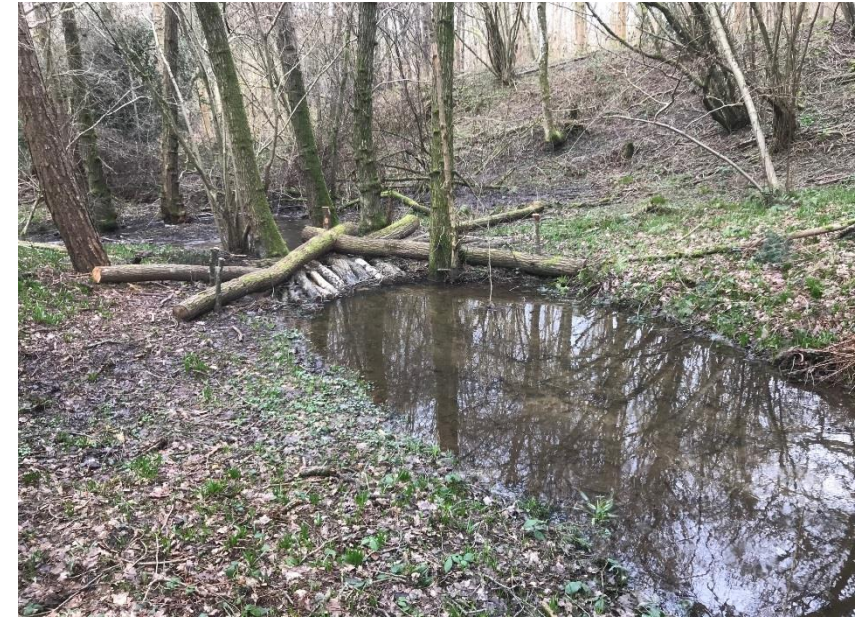
Leaky wood structure Alder Stream
